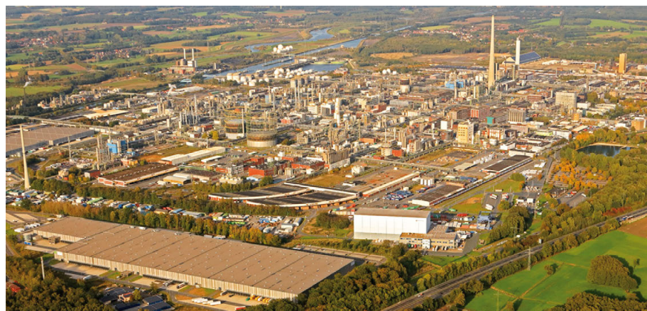
Fig. 1. Aerial view of Marl Chemical Park (CPM) [5] © Evonik Industries AG.
