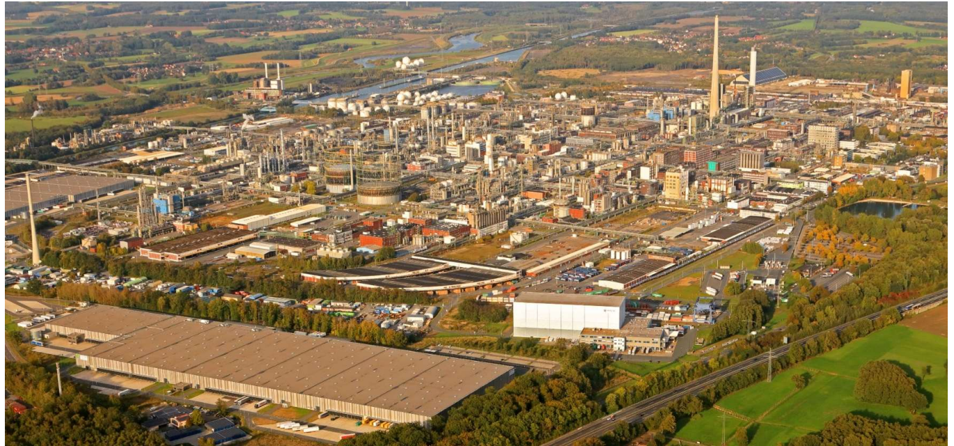
Aerial view of Marl Chemical Park (CPM) © Evonik Industries AG
